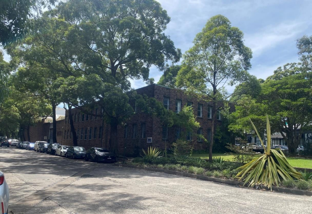
Figure 2: 242-258 Young Street, viewed from the south-west along Hunter Street, showing masonry building of 1-2 storeys
